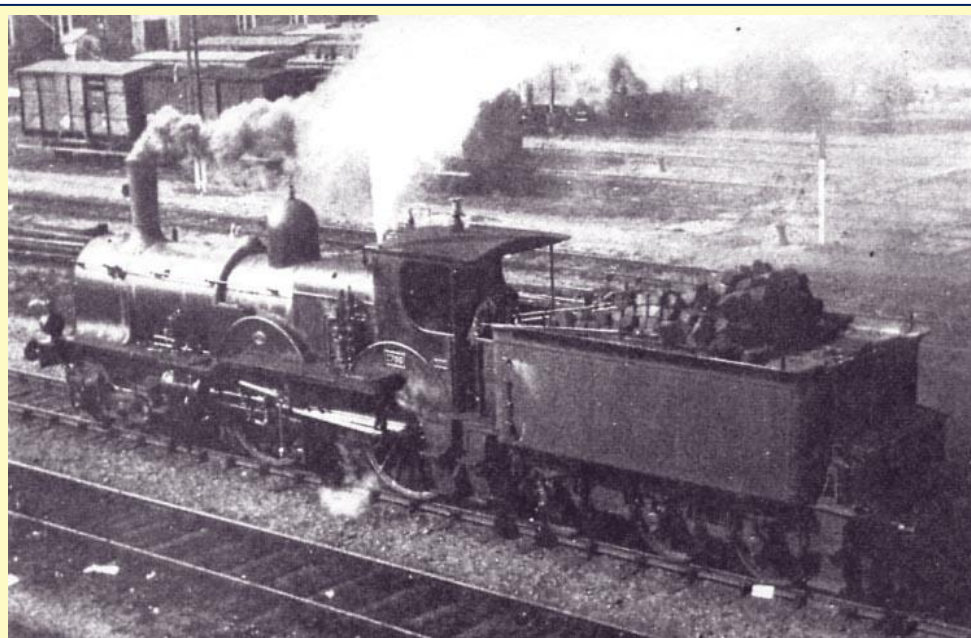
1894 - locomotive à grande vitesse, compound à 4 cylindres, série 1701 (Bordeaux)
